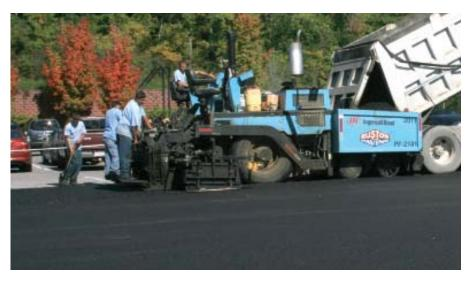
The entire recycled area was paved with two layers of hot mix asphalt,  $3\frac{1}{2}$  inches of binder and  $1\frac{1}{2}$  inches of top.
