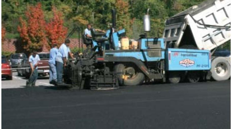
**The entire recycled area was paved with two layers of hot mix asphalt, 3½ inches of binder and 1½ inches of top.**
