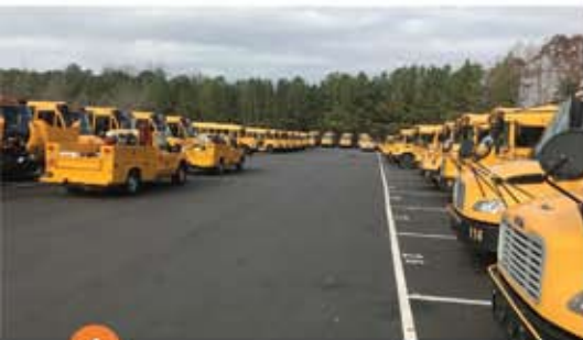
6 Completed pavement for the bus maintenance and storage facility.
